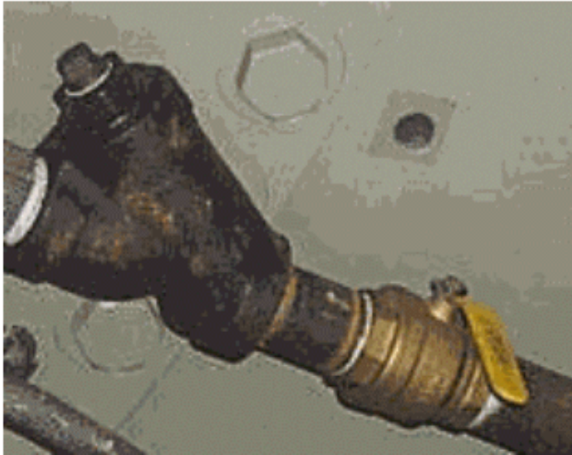
Figure 7. Flushing Filter Aligned to Preclude Oil Flow through the Filter when Removed for Inspection
