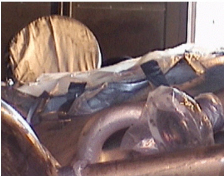
Figure 3. Examples of FME Covers utilizing Paper, Linen and Plastic Bags (Not a Recommended Practice)
